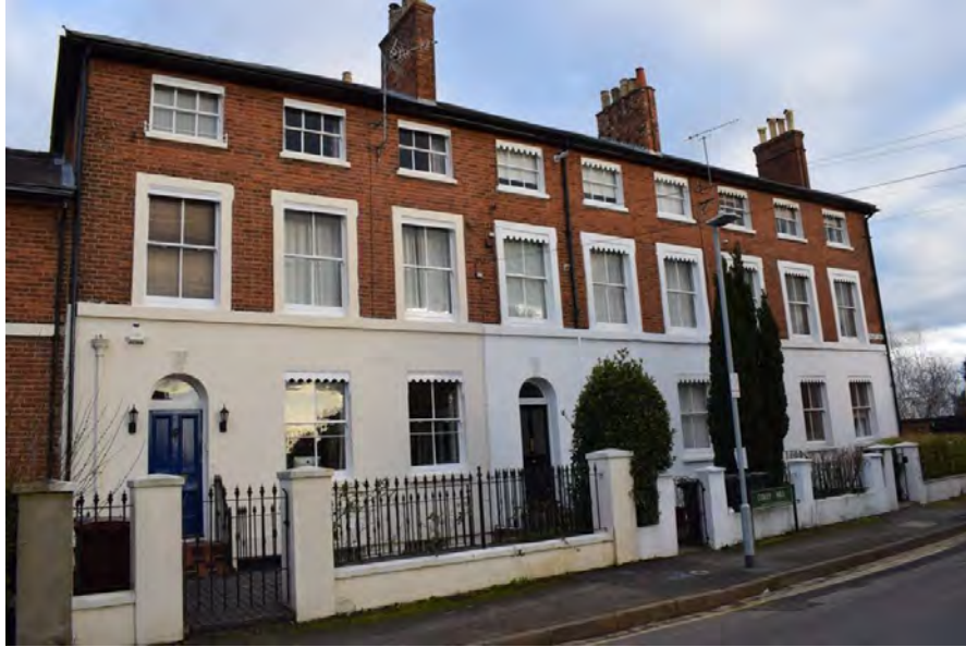
Figure 6.5.3 31-35 Coley Hill, stuccoed lower ground floor and later Victorian trimmed windows, 1820-30s (David Neale)
