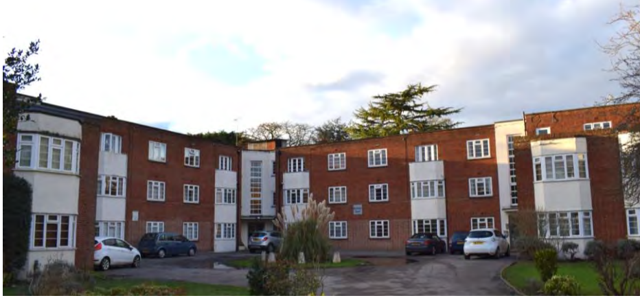
Figure 6.5.11 The mid 20 th century Berkeley Court, Coley Avenue (David Neale)
