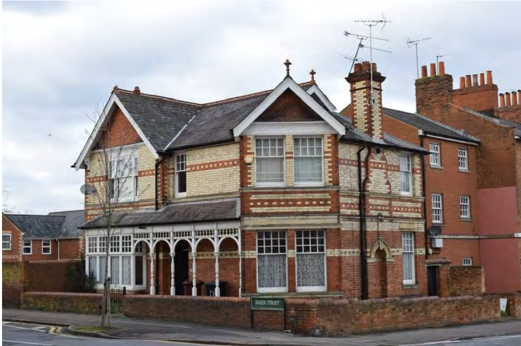
Figure 6.3.10 The Parsonage (c.1890) at the northeast corner of Baker Street and Russell Street with attractive polychrome and wood detailing (David Neale)
