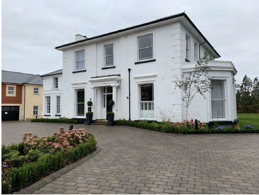
Figure 6.5.5 3 Castle Crescent after recent renovations (David Neale)
