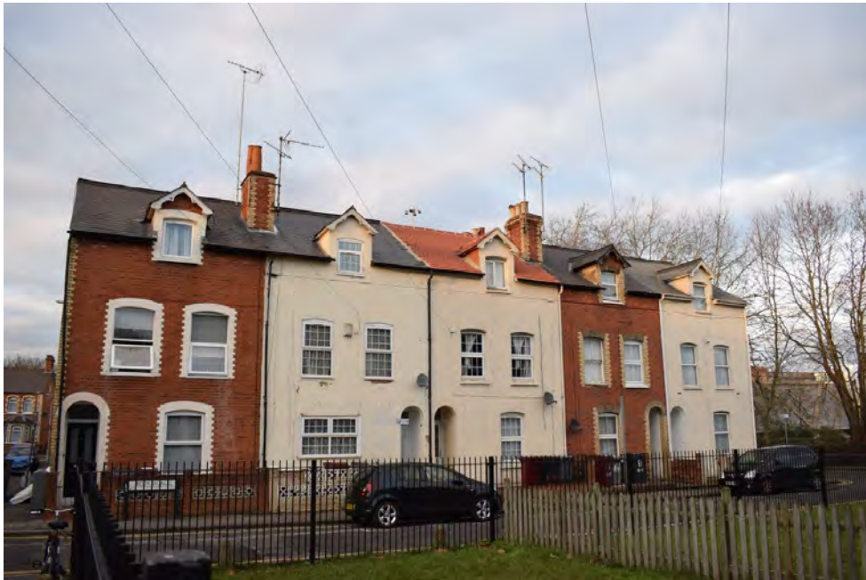
Figure 6.3.21 6-12 Body Road, the new red tile roof was installed in 2017 during the time protection of a conservation area did not apply (David Neale)
