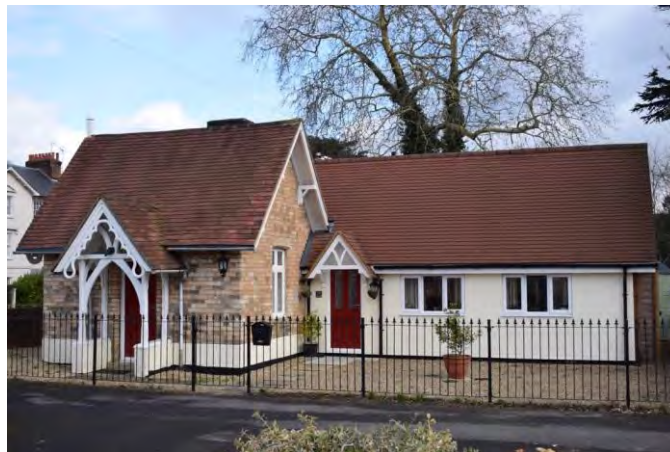
Figure 6.1.7 Former c.1840s gate house 133 Castle Hill for Yeomanry House, with the back section recently sympathetically built. (Karen Rowland)
