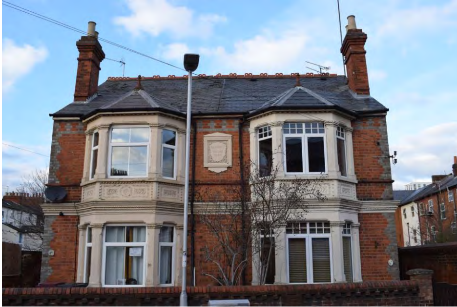
Figure 6.3.14 Rednirt Villas 1904, developed by Mr. Trinder, bay windows, polychrome and stone work detailing. Rednirt is Trinder spelt backwards. (David Neale)
