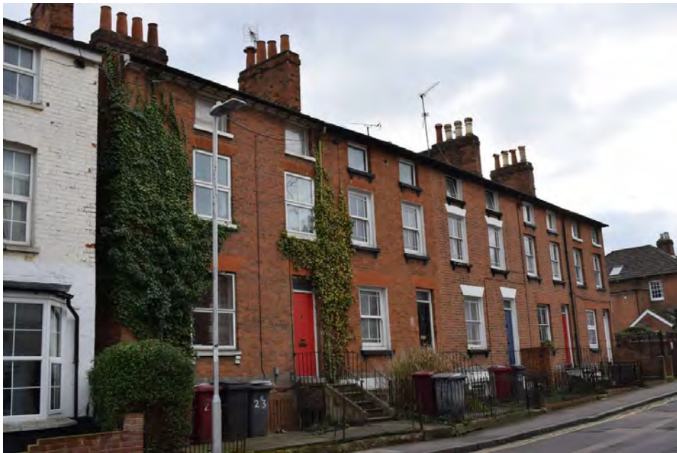
Figure 6.3.13 23- 31 Baker Street, Alexandra Terrace, c.1850, red brick terrace, overall well-preserved with majority of original windows and doors intact (David Neale)
