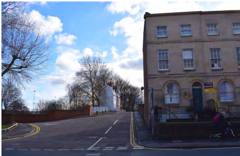
Figure 6.1.2 View 17: Looking south up Coley Place from Castle Hill (David Neale)
